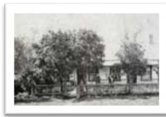
Brown House and Store, Route 307 near River Road (demolished)
